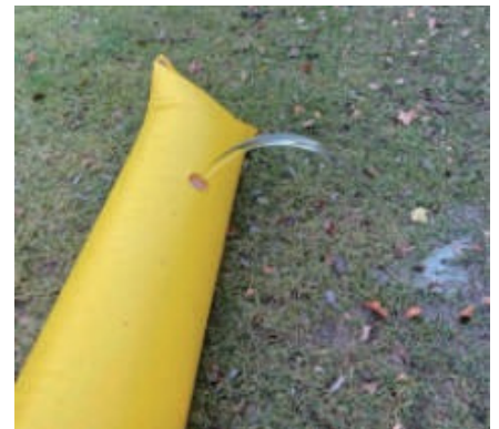
Drain the Tube After Flood Event
